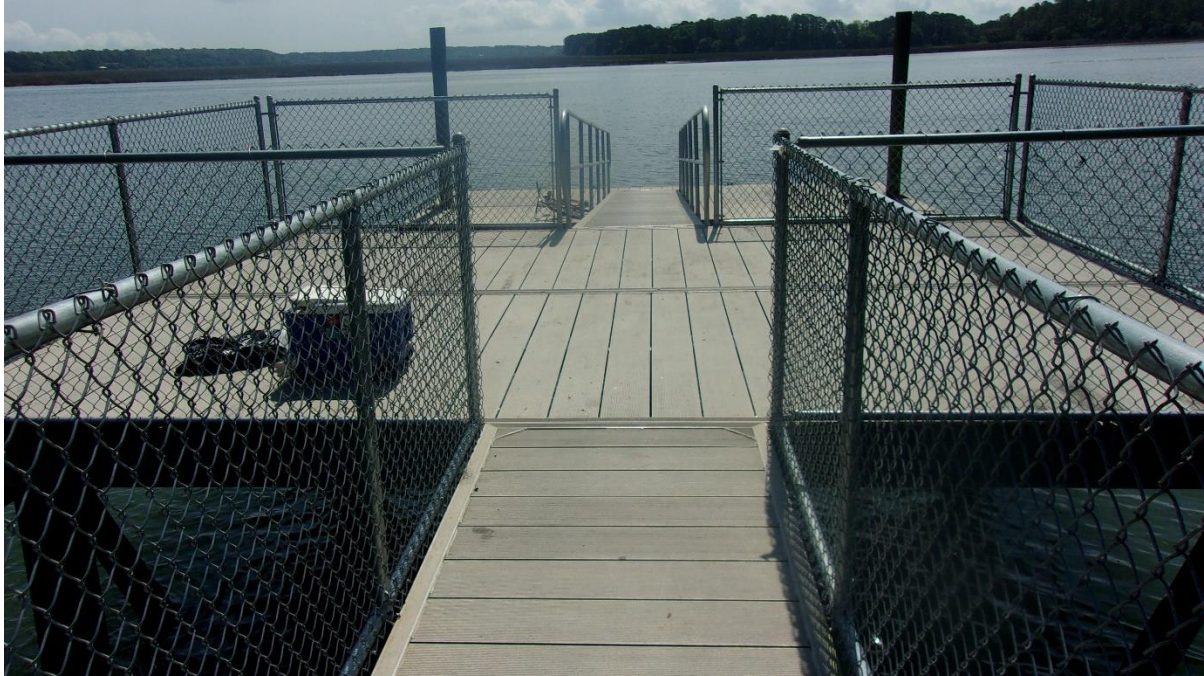
Dock, observed to be in good condition Note metal surfacing, aluminum railings
