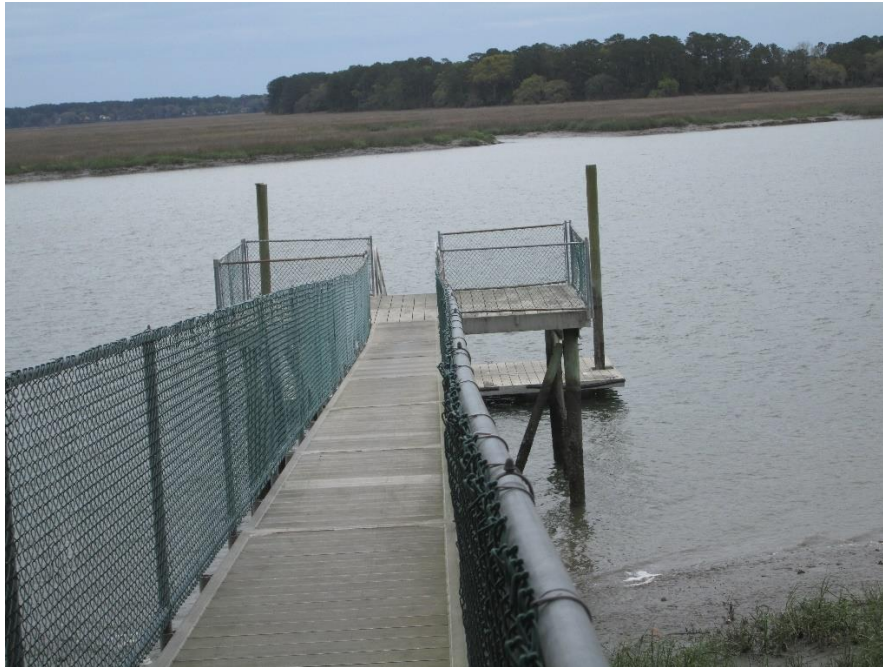
Dock, in good usable condition
